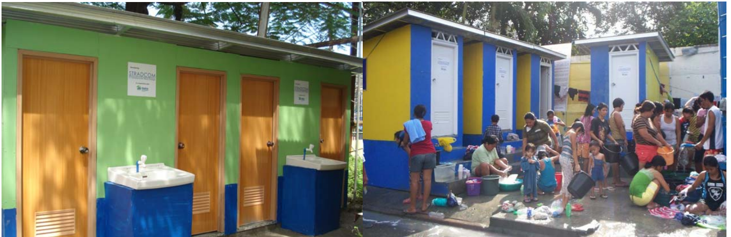
Sanitation facilities constructed by Habitat for Humanity Philippines and its volunteers, in partnership with Philippine National Red Cross and Stradcom Corporation. These pictured here are located at Bagong Silangan Elementary School, Quezon City (left) and Old Provincial Capitol, Pasig City.
