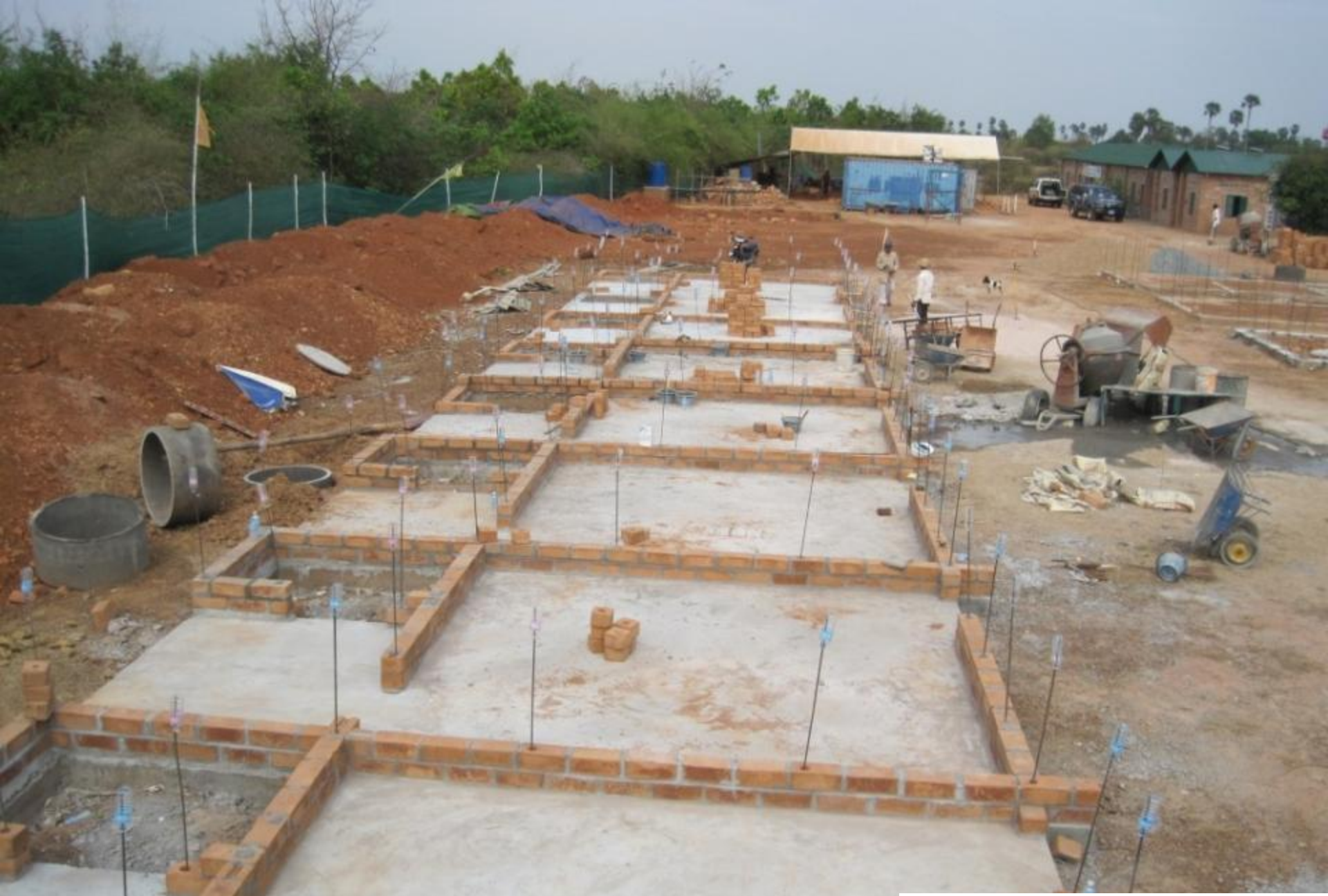
Build site: row house foundation floor
