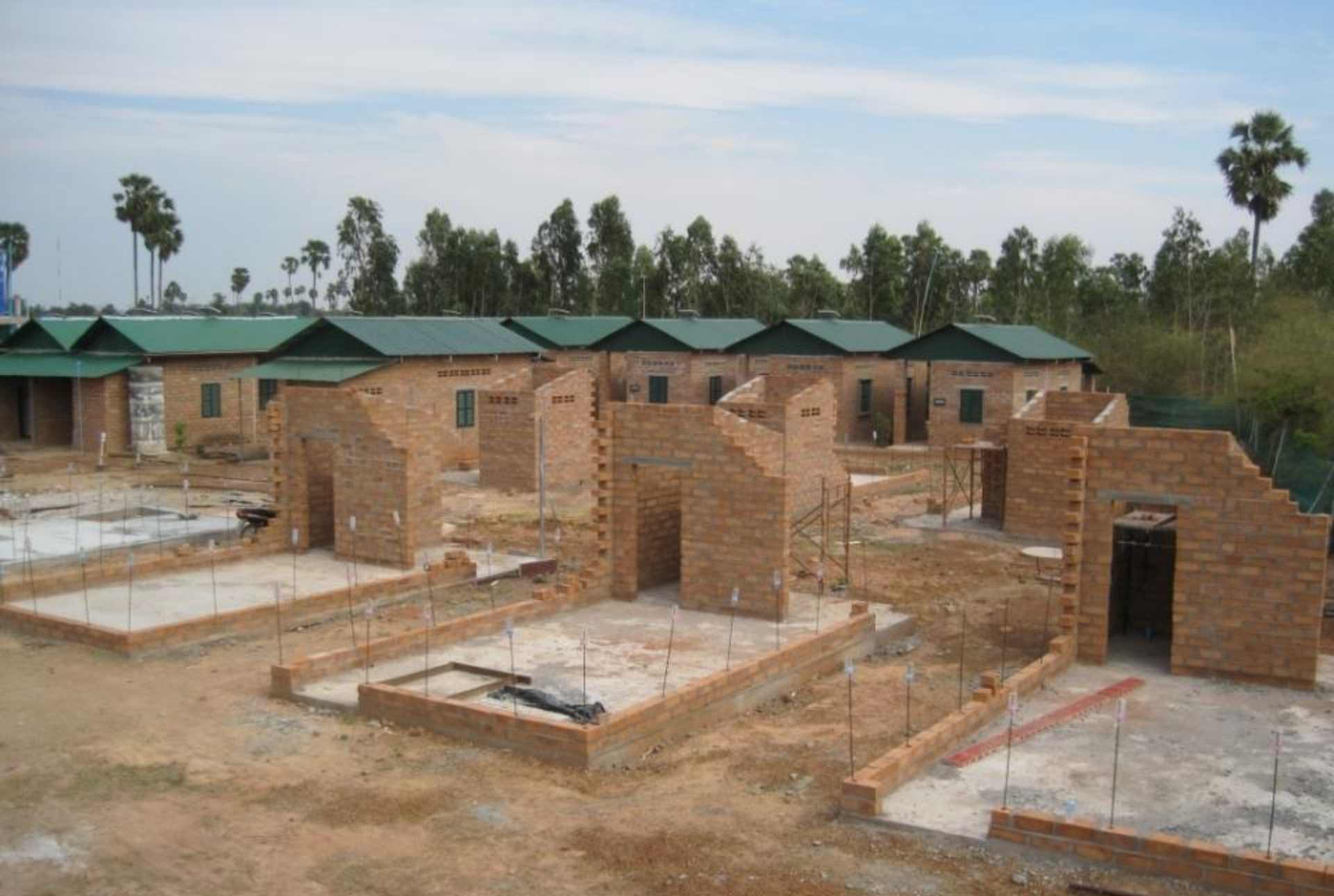
Build site: Single detach house foundation floor
