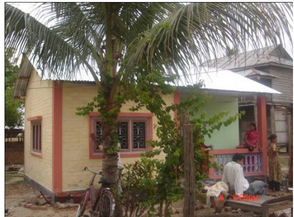
294 Sq.ft. house, stone and concrete foundation Concrete pillar
