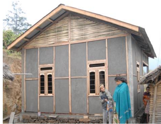
330 Sq.ft.house, Stone foundation, Bamboo wall plastered with cement
