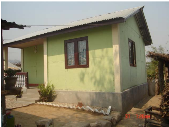
(280 Sq.ft. house, stone foundation, Bamboo wall in timber frame with cement plaster and tin sheet roof)
