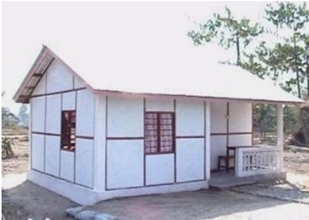
(280 Sq.ft house, Stone foundation, Bamboo wallplastered with cement
