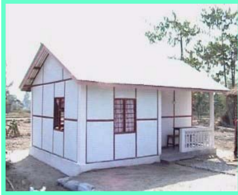
Completed house in Nepal with the use of bamboo technology
